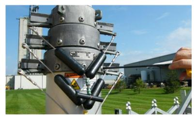
Figure 3-1 Remove One Collar Bolt and Washer from Bottom Section Collar
