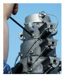
Figure 3-7 Remove One Collar Bolt from each Collar
