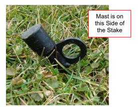
Figure 4-30 Drive Each Stake into the Ground at a 45° Angle
