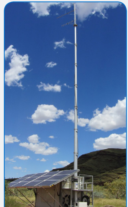
Locking Pneumatic Mast
