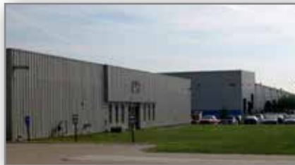
Manufacturing | Orrville, Ohio
